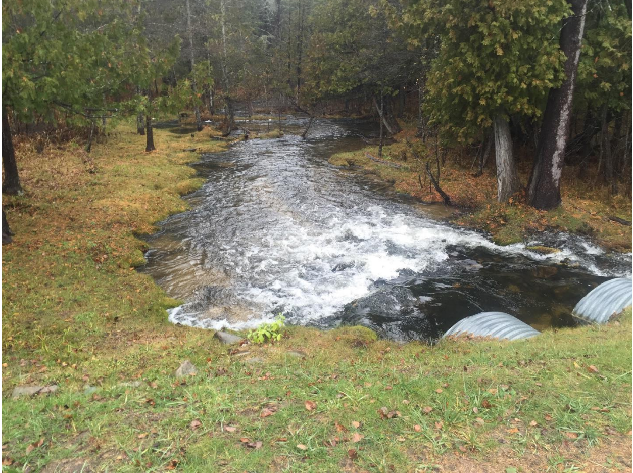
Figure 7. Downstream side of the Finch Creek Rd crossing of Finch Creek
